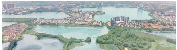
Rasau Water Supply Scheme Phase 1 (700 MLD capacity)
